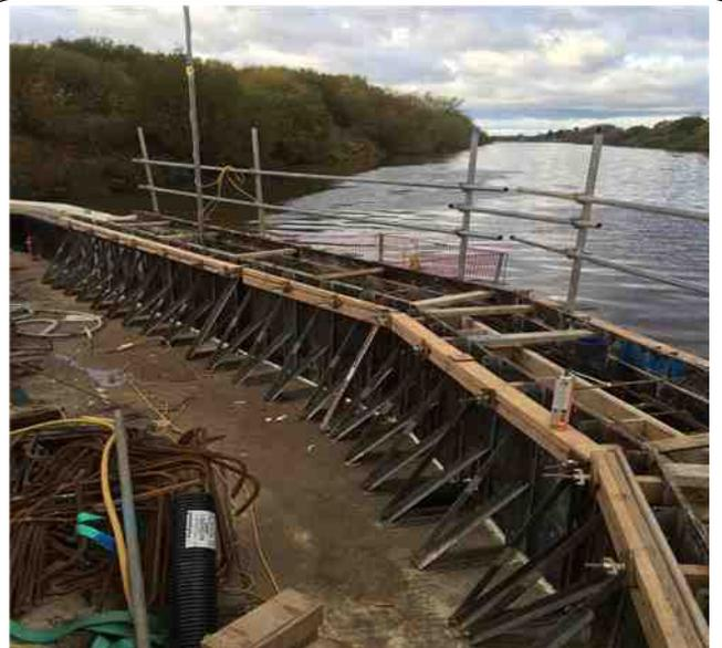
**Cross rail capping beam (3m drop on other side)**
