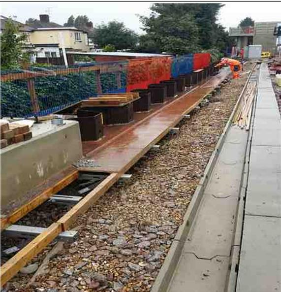
**Capping beam with angles and mix of land and river sides**
