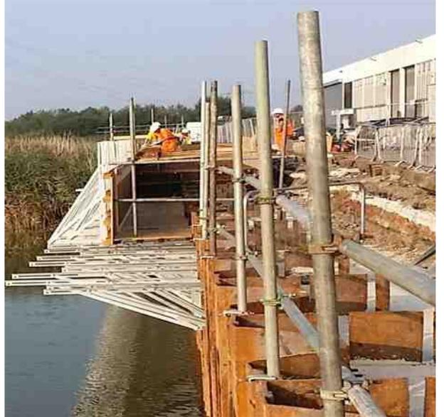
**Small capping beam to Railway embankment**
